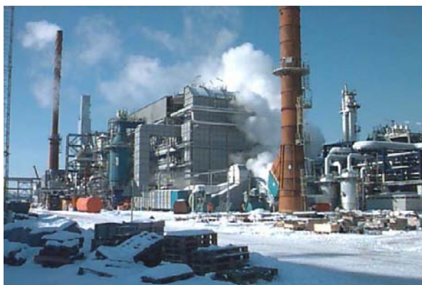
Figure 21: Synthesis gas plant of 2,500 MTPD methanol plant, Statoil, Tjeldber-godden (Source: HTAS)
