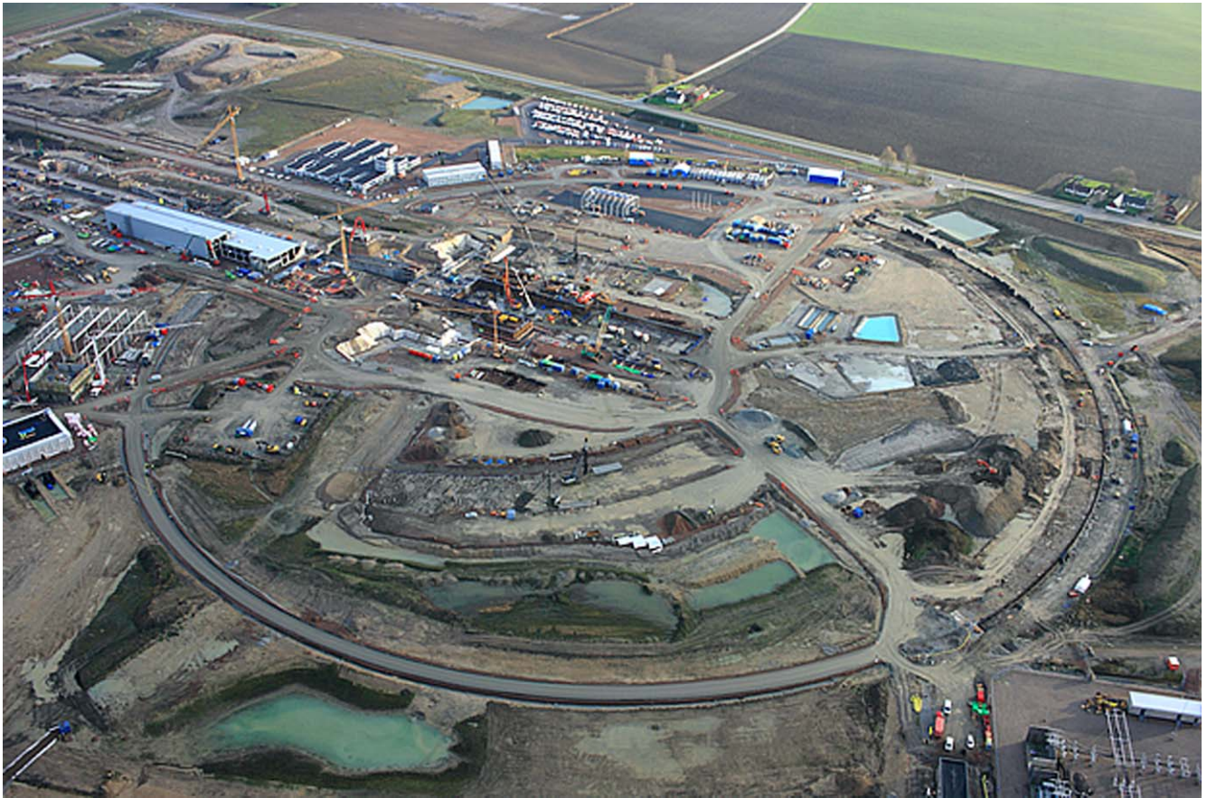
Figure 112. Aerial view of the ESS construction site, July 2016.
