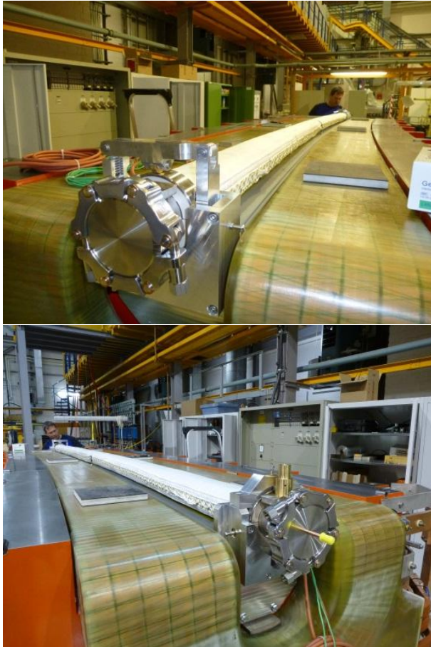
Fig. 38: Dipole chamber with heating jacket during installation inside the dipole magnet.
