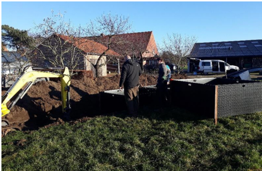
Figure A6. Excavation works during set up of experimental site, showing the black impermeable plastic boxes and the crane used for de-compaction.
