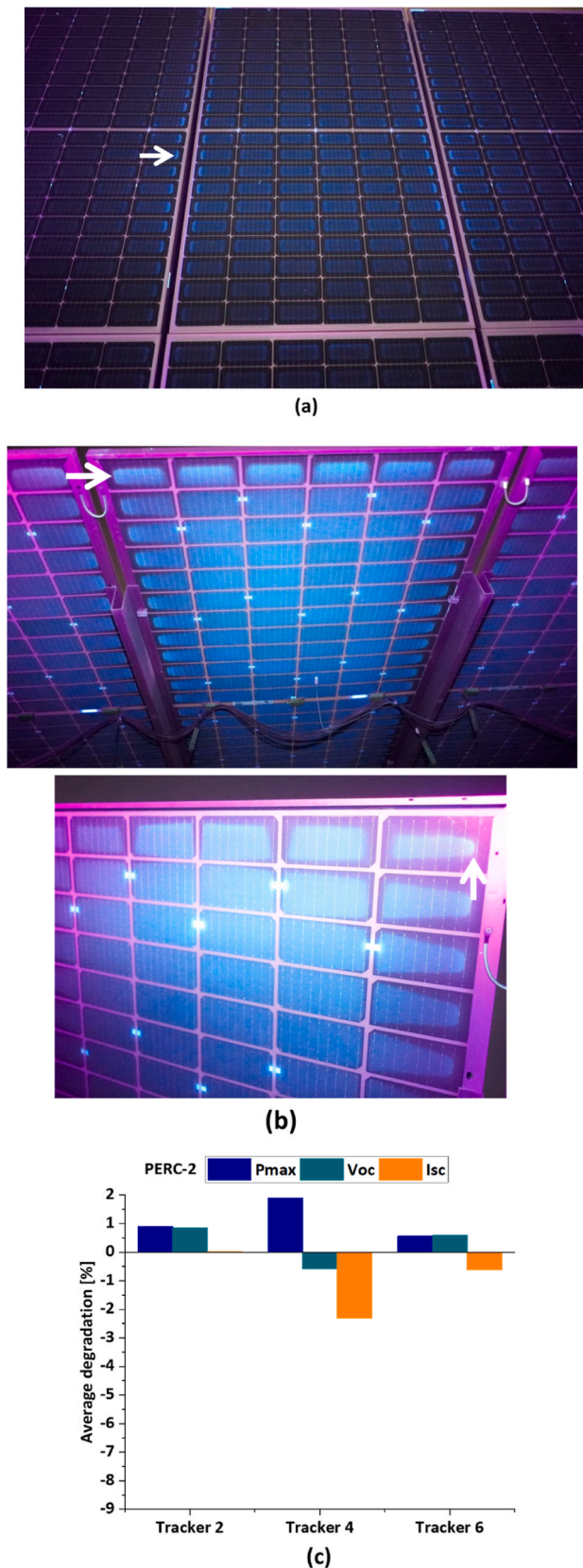
Fig. 4. Early degradation in bifacial PERC-2 PV modules with framed glass/glass configuration installed on trackers 2, 4, and 6: (a) UVF degradation pattern of the front side indicated by an arrow, (b) UVF pattern on the rear side indicated by an arrow, and (c) variations in the average measured electrical parameters P_{max} , I_{sc} , and V_{oc} .
