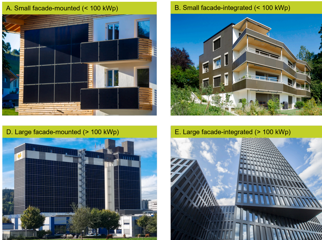
Fig. 1. Exemplary solar facades. A. small facade-mounted (<100 kW) [79] B. small integrated (<100 kW) [80] C. large facade-mounted (>100 kW) [81] D. large integrated (>100 kW) [82].
