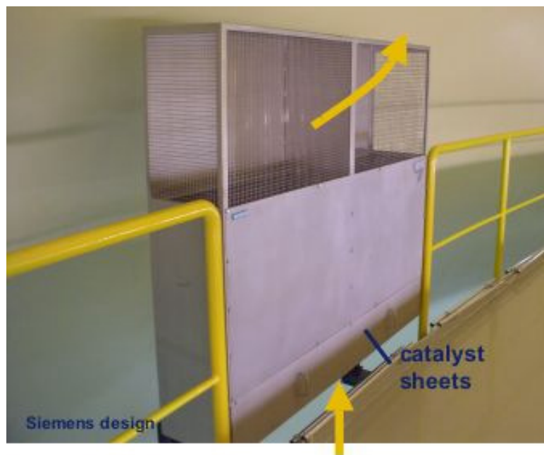
Figure 8-24. Principle of a passive catalytic recombiner
