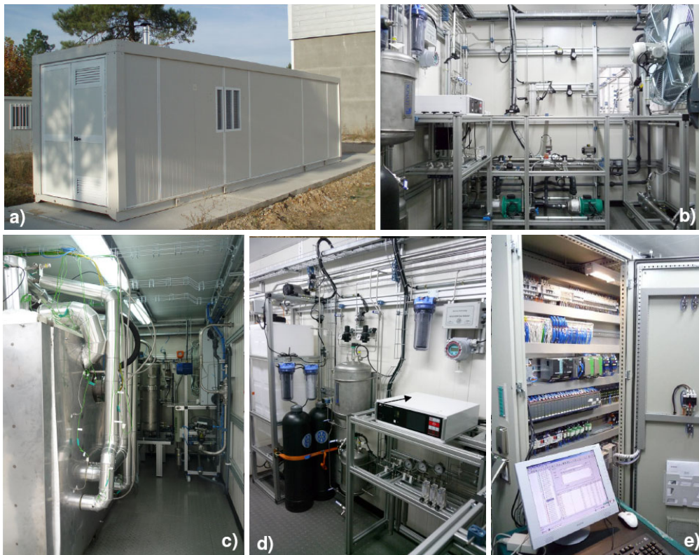
Figure 4: Fuel processor facility; a) Exterior view of the cabinet, b) Instrumentation of feeding lines and cooling of the reformer, c) set of reactors and scrubber, d) Gas measurement systems and water line, e) electric enclosure and control system.
