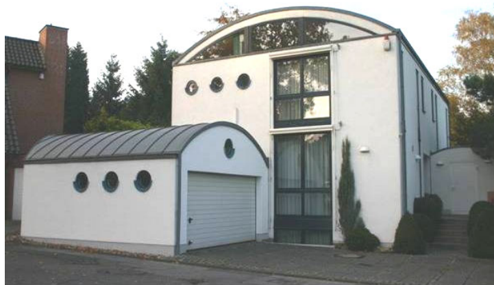
Figure 5: Single-family home in Mülheim/Ruhr, Germany, with Galileo 1000 N [Source: T.B.E. GmbH, Duisburg].
