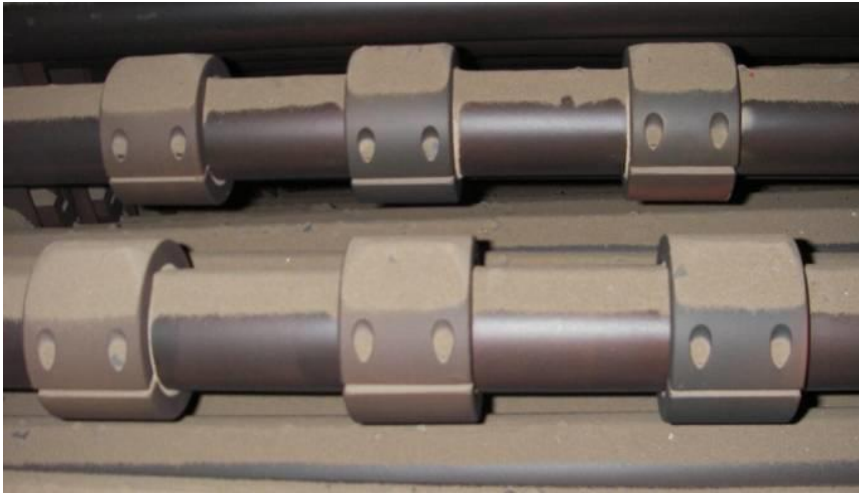
Figure 9: Evaporator inlet clamp and INTREX clamps
