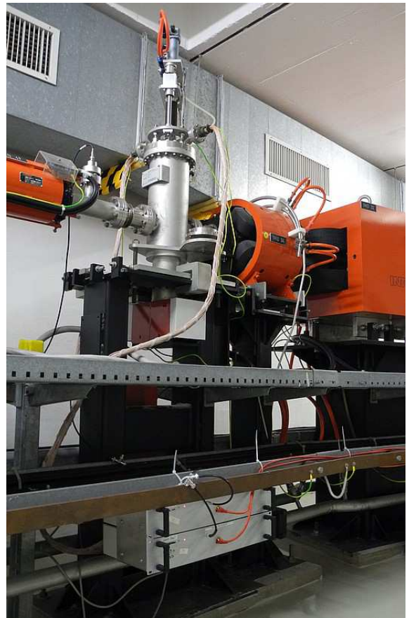
Fig. 2: PG4.1 in the COSY IBL. Below the cable duct the new readout electronics is installed.
