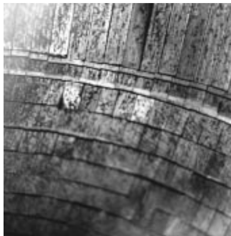
Figure 1. View of the inner wall of the Extrap T2 vacuum vessel after thousands of plasma discharges, with full coverage provided by small graphite tiles. Some imperfections in the alignment of the tiles and damage to the tile edges are visible.
