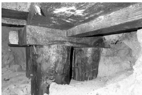
Figure 4: Excavated foundation piles in Amsterdam (Photo: Fugro).
