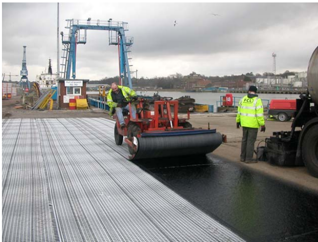
Figure 39: Reinforced asphalt overlay (glass reinforced fibres) at Ipswich Docks, RoRo Ramp, (photo with kind permission from www.asphalt-geotextiles.co.uk )
