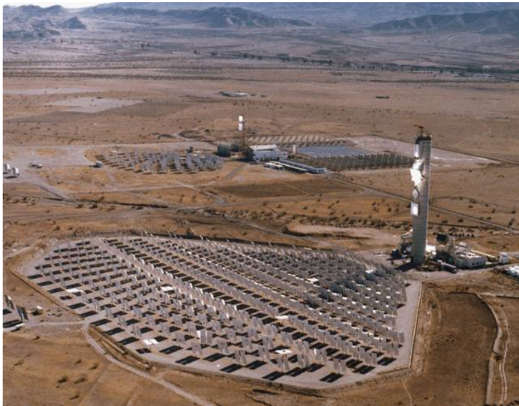
Figure 23. Solar Thermal Central Receiver Systems (SIREC) 58 : In this plant in Andalusia, Spain, a high-flux receiver ( 2 \text{ MW/m}^2 ) has been installed, which has a compact design and a ceramic absorber. This device operates at temperatures of 1000 \text{ }^\circ\text{C} and has a self-regulation system to adjust air recirculation flow rates.
