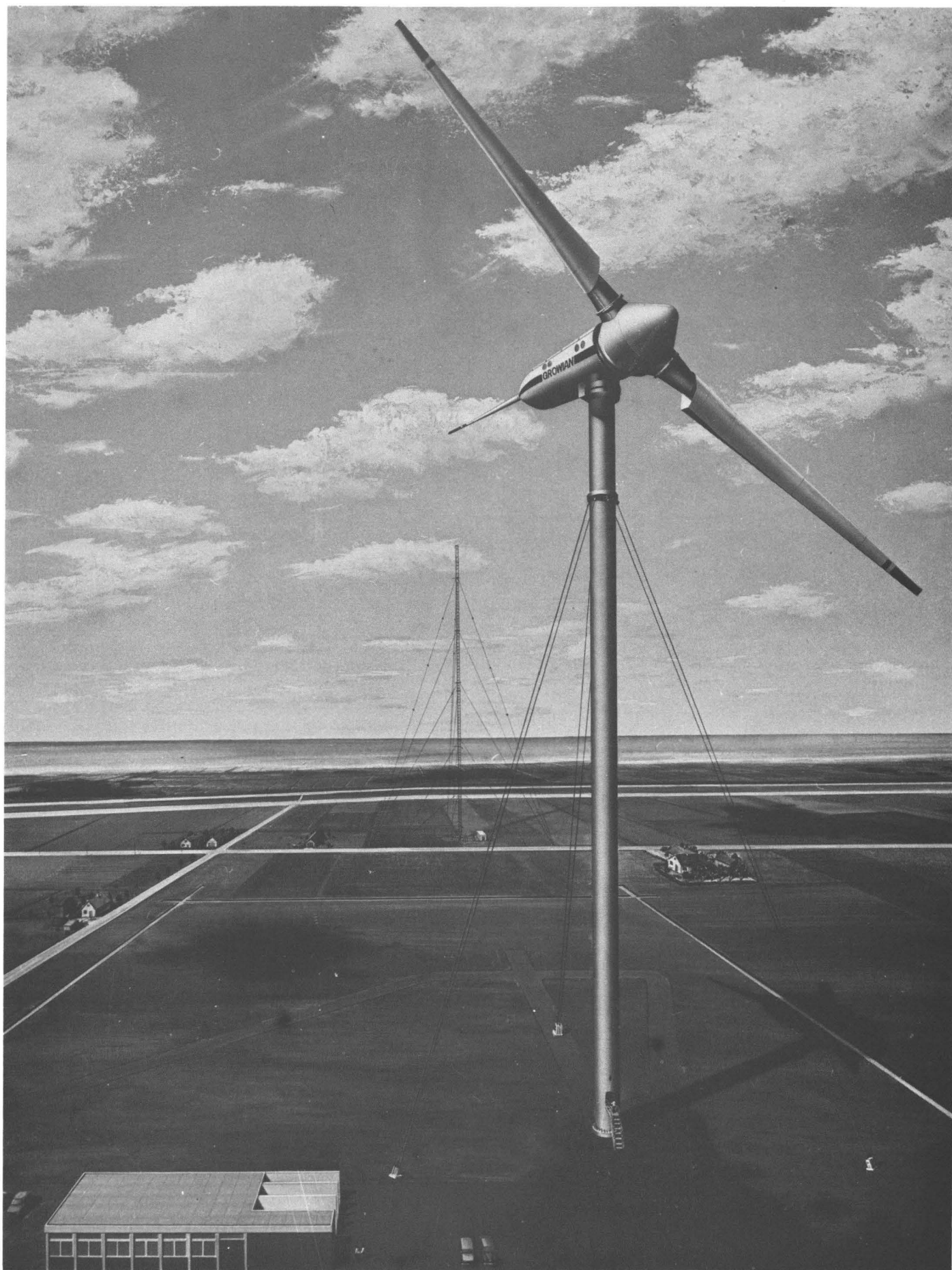
The German LS WECS GROWIAN: 3 MW from 12 m/sec up to 24 m/sec wind velocity, Kaiser-Wilhelm-Koog, mouth of the Elbe. View to SW in main wind direction. First rotation autumn 1982.
