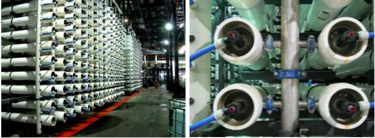
Figure 1. Views of a desalination reverse osmosis plant such as the Ashkelon Desalination Plant in Israel showing stacks of RO-membranes. Such a plant produces of the order of 500,000 m 3 potable water per day.
