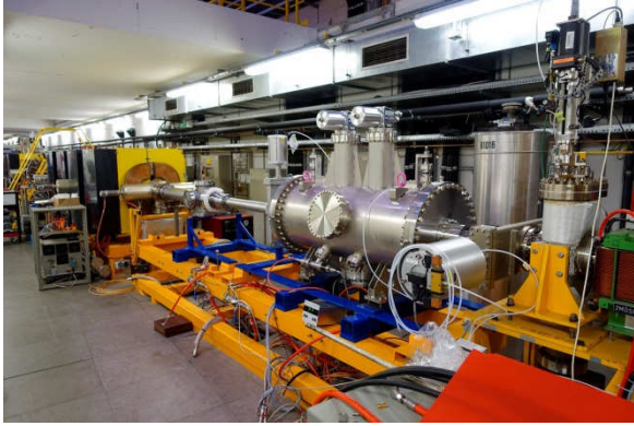
Figure 2: Installation of first HESR pickup tank in COSY.
