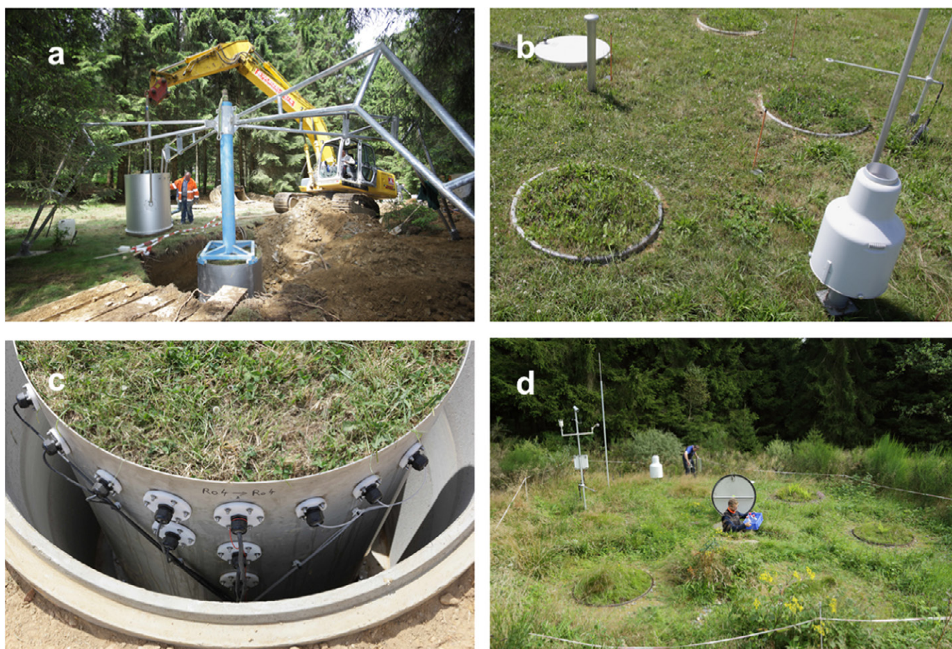
Fig. 2. (a) Coring of an undisturbed lysimeter core, (b) installed lysimeter, (c) instrumentation, and (d) view of a lysimeter setup with underground access.
