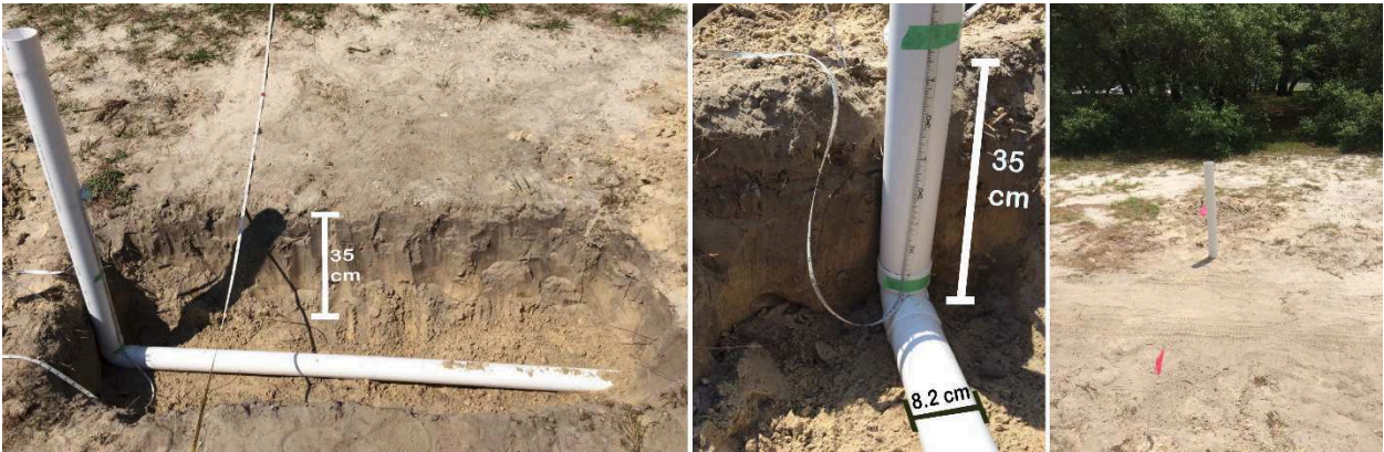
Figure 7. Left, the L-shaped PVC pipe in the hole in sand. Middle, the elbow part of the pipe showing the burial depth of 35 cm for the top of the horizontal part. Right, after filling the hole, the vertical part is visible that enables filling the pipe. The horizontal part of the pipe is aligned between the pink flags.
