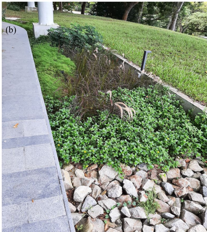
Fig.1. Schematic showing different components of a typical field-scale stormwater bioretention cell (a), and image of a bioretention facility installed at National University of Singapore.
